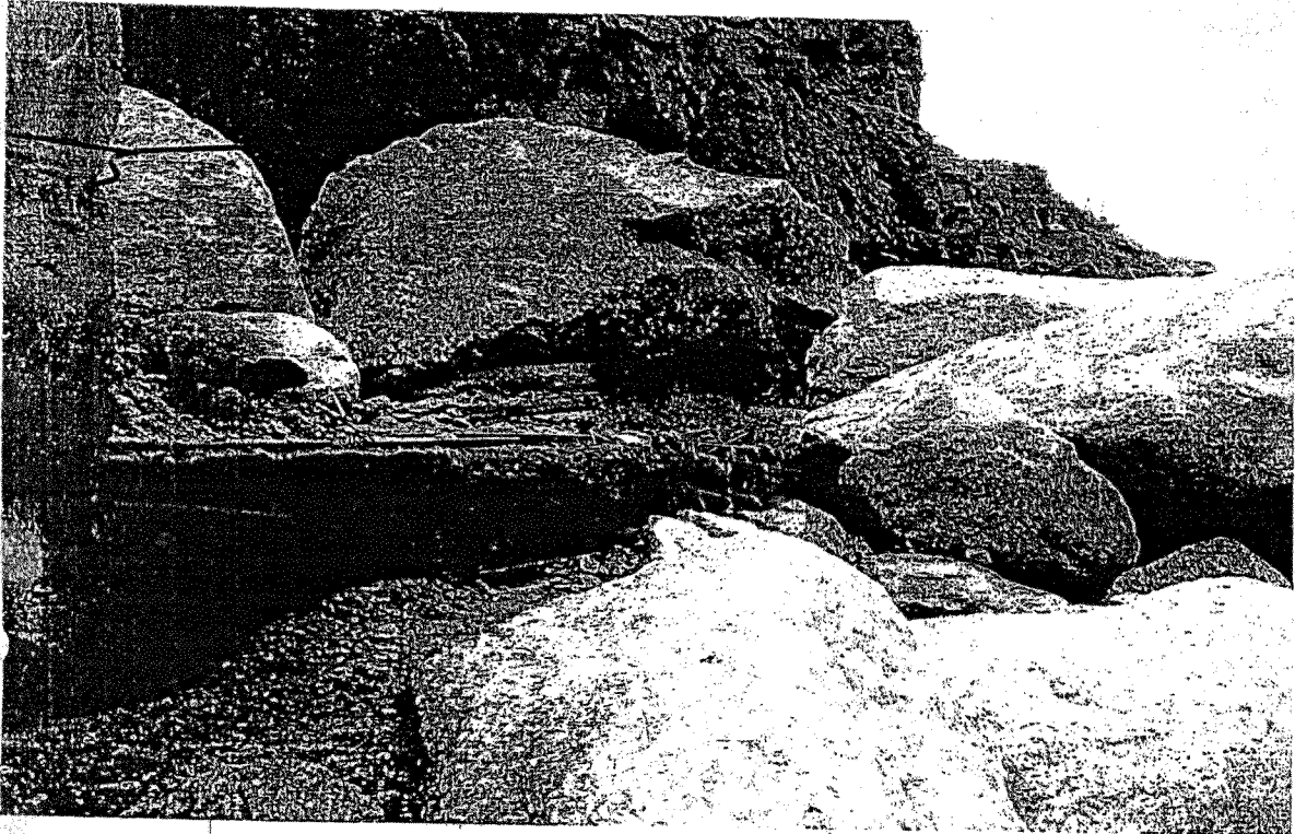
Deserting chamber after cloud burst (Big boulder coming in D-TANK)
