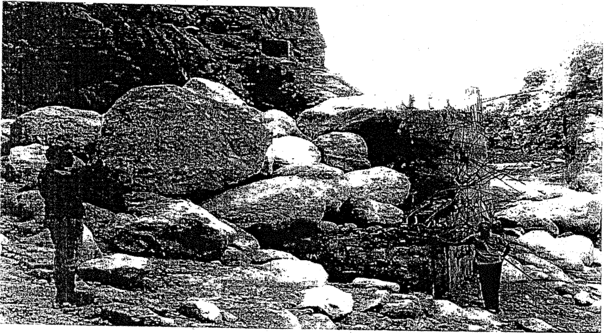
Desilting chamber after cloud burst (Big boulder coming in D-TANK )
