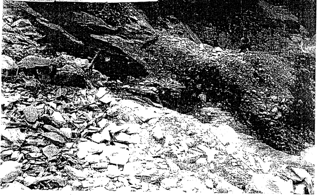
Road Damage during Rainy season July, Aug Sep 2008
